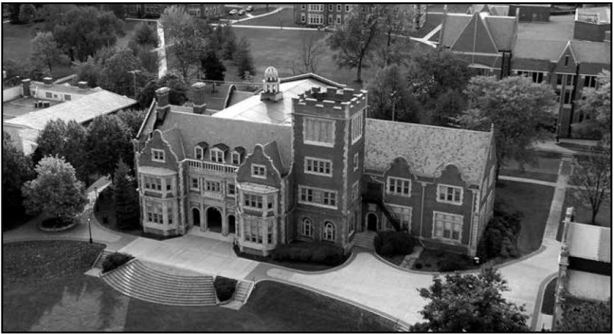
Aerial view of the campus, ca. 2005
