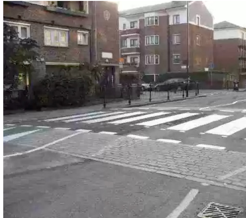
Image 2: Continuation of Pedestrian Surface across Roadways in Copenhagen, Denmark. Cally Labour Councillors, 2010.
