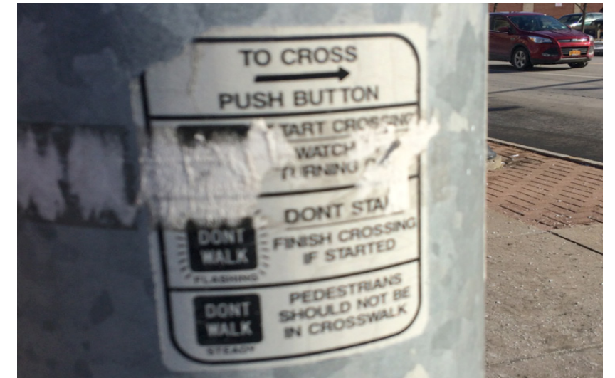
Image 8: Peeling Crosswalk Signage
